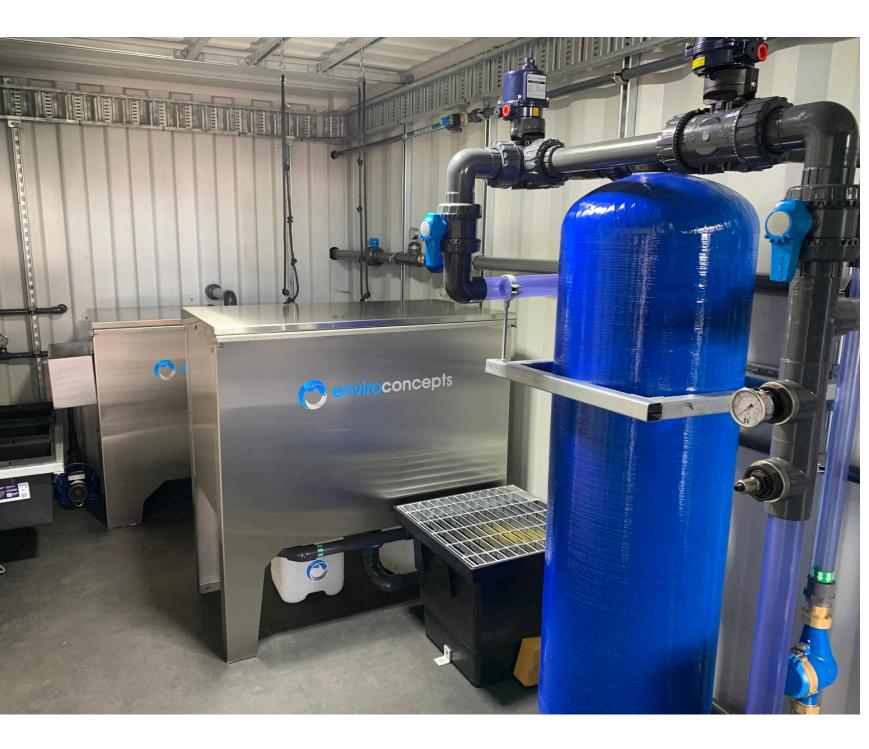
Water Recycling System | 30 to 100 L/min
